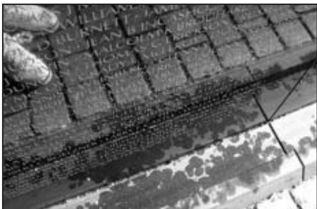
The names along the lower part of The Wall appear to have taken the brunt of the damage.
